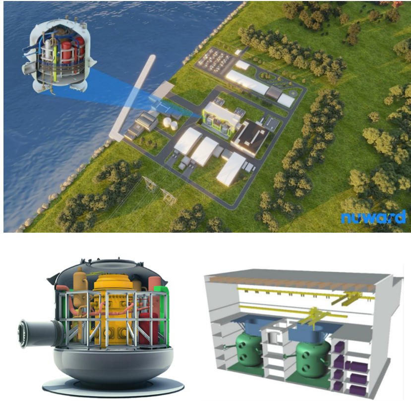
Figure 4.1.1: Presentation of NUWARD™ project and its design principles, a 340MWe SMR plant with two independent reactors (170MWe each) housed in a single nuclear building
